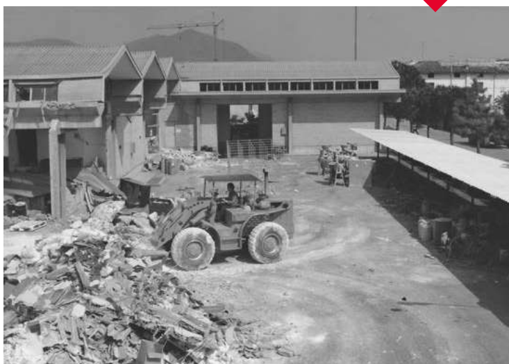
Ledraplastic plant during post-earthquake reconstruction (1976)
